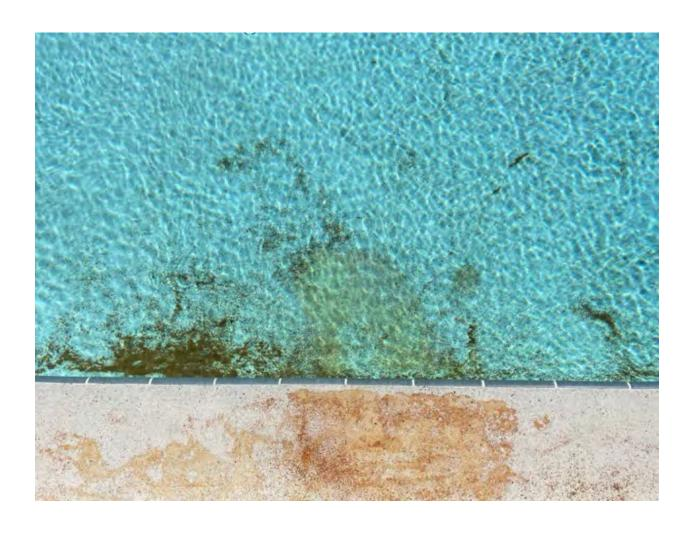
Pool damage caused by a leaking handicap chair battery.
