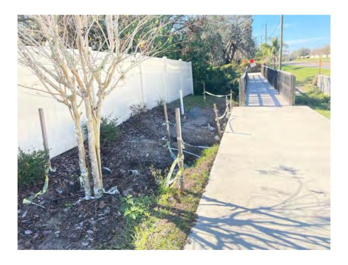
The washout next to the 14<sup>th</sup> Ave SE sidewalk has not been repaired.
