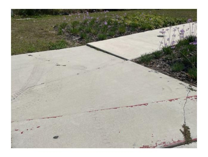
There is a crack in the sidewalk, & the curbing is raised on the East Golden Glow sidewalk.
